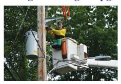
Georgetown Light continues to upgrade its infrastructure to meet the needs of its customers with the conversion of a 4 kV distribution line to a 13.8 kV line in the Lakeshore Drive area. The conversion will increase system capacity and enhance reliability as customer needs change due to rapid technology advances and increasing demand.
