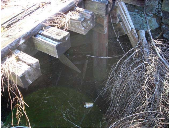
Figure 6: Bridge No. 164 Existing Timber Pile Bents
