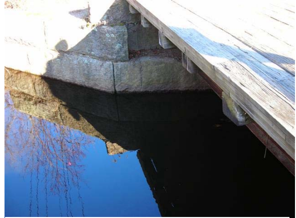
Figure 11: Bridge No. 166 Existing Granite Abutments
