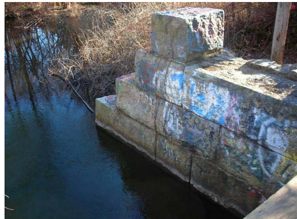
Figure 9: Bridge No. 165 Existing Granite Abutments
