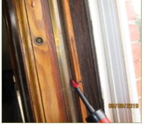
Right: Town Hall – smoke testing along the wood, double-hung windows indicates air-leakage, partly due to some shrinkage in the wood framing, but mostly due to failing or missing weatherstrip. New weatherstrip (including sash locks and pulley seals) needs to be installed on the wood-framed and metal-framed windows basement sections.
