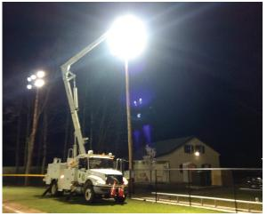
Georgetown Municipal Light Department recently installed fusing on lights at the Penn Brook School ball field. The new lighting system will be more reliable, enabling crews to pinpoint the source of any problems and eliminating the need to check each light and running the risk of ruining the field.
