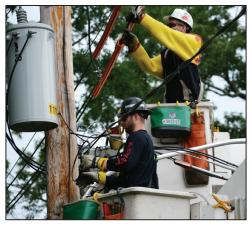
Georgetown Light has completed the conversion of a 4 kV distribution line to a 13.8 kV line in the Lakeshore Drive area. The conversion involved the tying together of two circuits to increase system capacity and enhance reliability as customer needs grow due to rapid technology advances and increasing demand.
