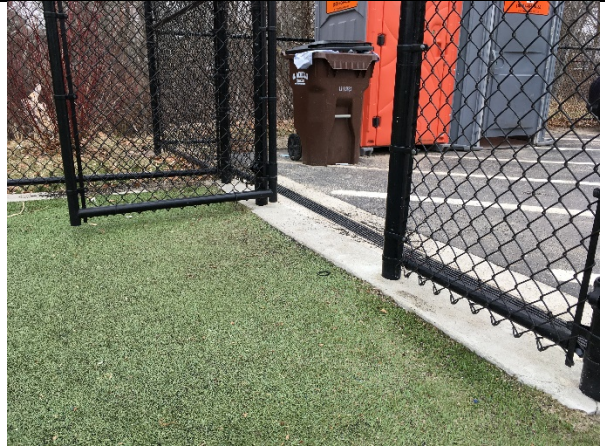
Trench drain in concrete transition at primary access entryway.
