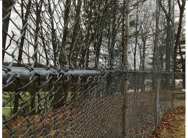
Backstop fencing damaged and showing signs of rust.
