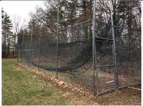
Chain link batting cage showing structural damage and loose protective netting.
