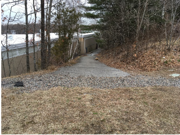
Paved access to field is significantly sloped, ADA non-compliant.
